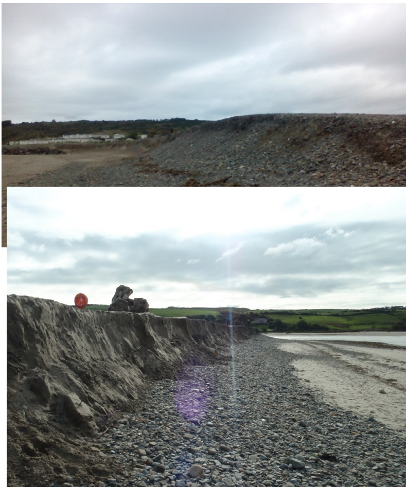
Fig 9. 02/10/2018 Pen yr Eryd Spit. Erosional scarp in the reconstructed upper spit two weeks before. 7.5m wide crest reduced to 4m at the distal end.
