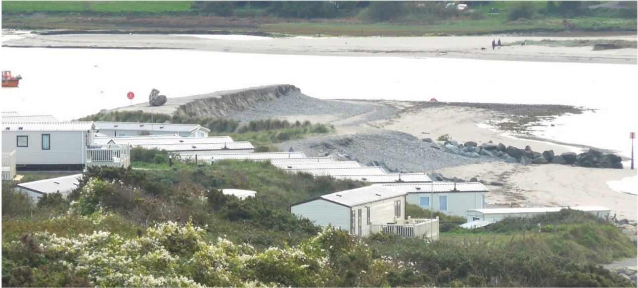
Fig 8. 16/10/2018 Pen yr Eryd Spit. Note the engineered upper surface ~5.2m OD. The near vertical erosional scarp along the reconstructed upper crest. Although this is post storm Callum there is no evidence of over-run or debris flows on the inner slope. The large feature on the spit crest is a tree root place there by the ATFL. Source: Chris Evans.
